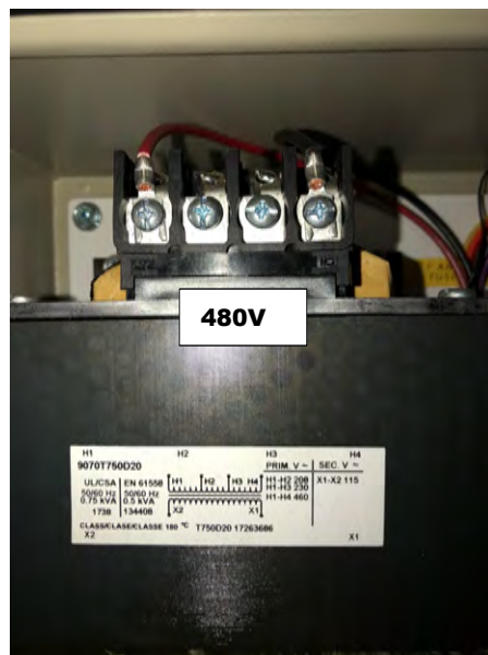
480V 3PH ONLY MODELS TRANSFORMER PRIMARY WIRING
