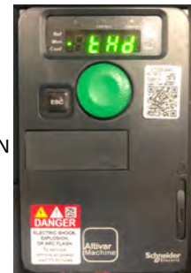
DRIVE THERMAL STATE 100%=NORMAL 118%=OHF THRESHOLD
