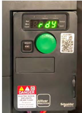
VFD DISPLAY (NEW VERSION ATV320)
