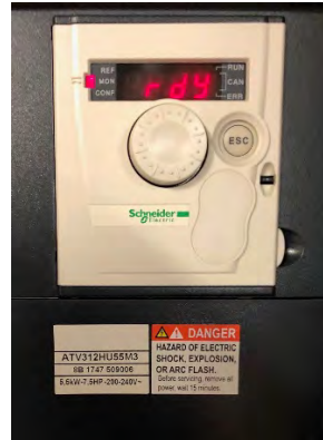
VFD DISPLAY (PREVIOUS VERSION ATV312)
