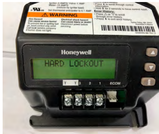
HARD LOCKOUT AFTER A FAILURE TO PROVE FLAME IN ALLOCATED 15 SEC. TRIAL FOR IGNITION PERIOD OR OTHER FAILURES SUCH AS FLAME PRESENCE PRIOR TO IGNITION TRIAL. RESET BY REQUIRED BY PRESSING "i" BUTTON FOR 2 - 3 SECONDS AND RELEASING. A MAXIMUM 3 RESETS CAN BE ATTEMPTED.
