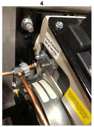
Place splined nut in safe location such as on fuel line tube.
