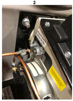
Move copper fuel line tube away from burner
