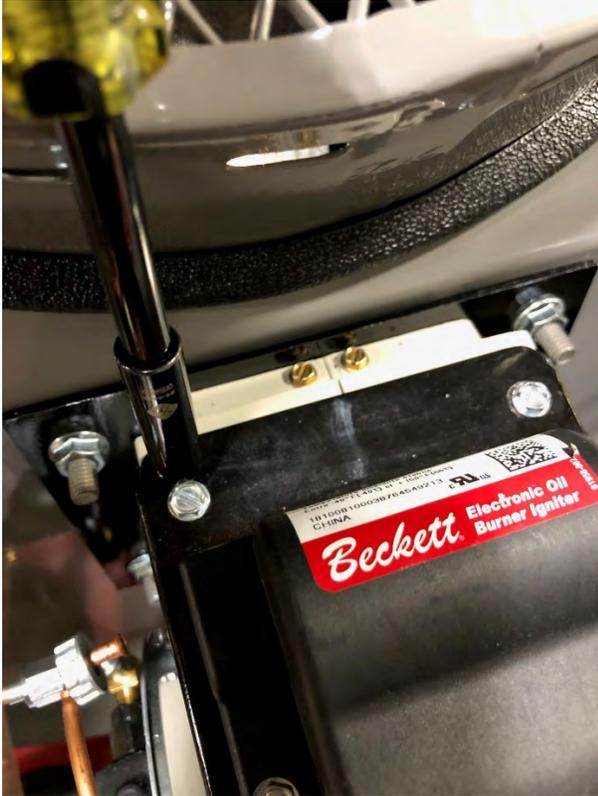
Remove ignitor retaining screws with 5/16" socket or wrench.
