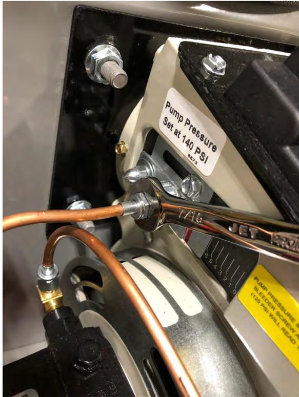
Remove fuel line connection from burner inlet.
