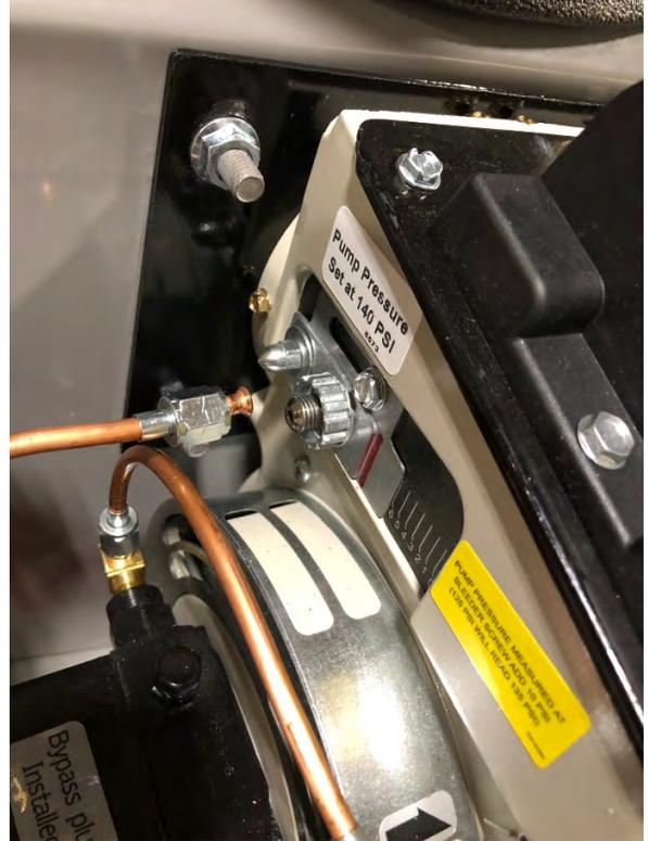
Move copper fuel line tube away from burner
