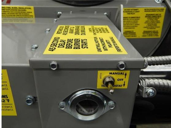
Figure 1: Front two screws to remove
