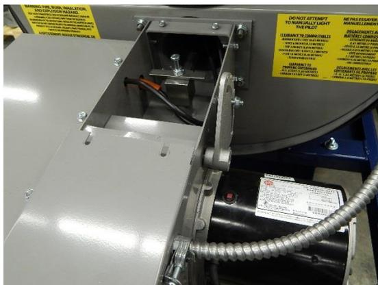
Figure 3: Sliding the burner access cover off
