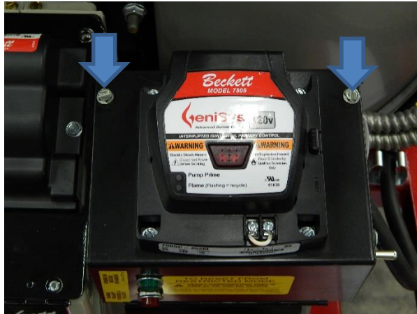
Figure 3: Controller cover with fasteners indicated
