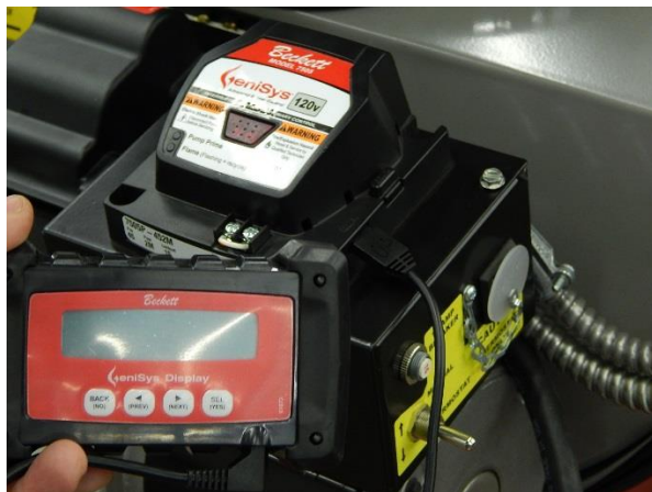
Figure 2: Genisys contractor tool attached to controller
