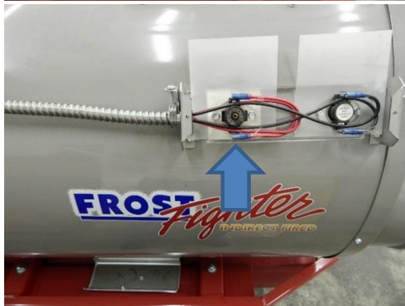
Figure 1: Fan switch cover near front of unit
