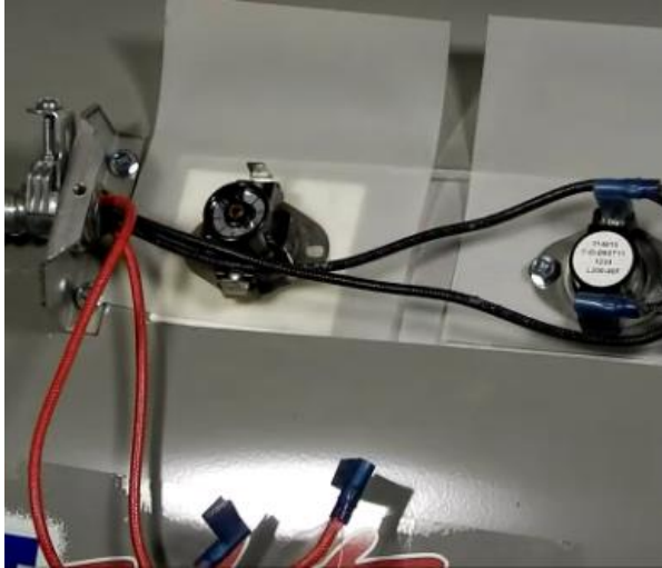
Figure 3: Fan switch which is ready to be removed
