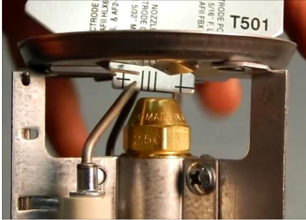
Figure 2: Loosening fasteners to position electrode
